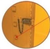
Welded shelf hangers interlock with shelf to offer maximum "no slip" stability.. And no flimsy brackets to lose.
